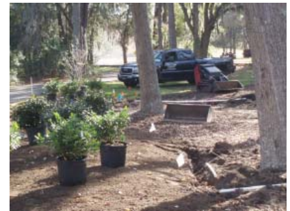
Palmetto Coastal Landscaping is at work on this project.
